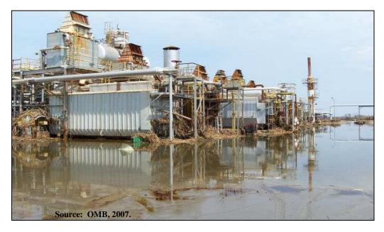
Figure 89. Natural gas processing plant flooded by Hurricane Katrina.
