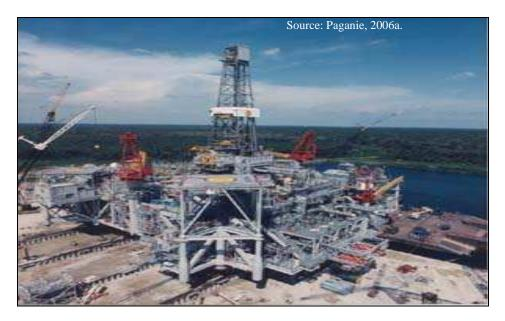
Figure 10. Independence Hub's topsides under construction at fabrication yard near Corpus Christi, Texas.
