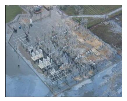
Figure 137. Substation flooded by Hurricane Katrina.
